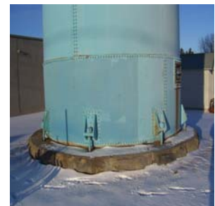
Note the limestone block foundation
